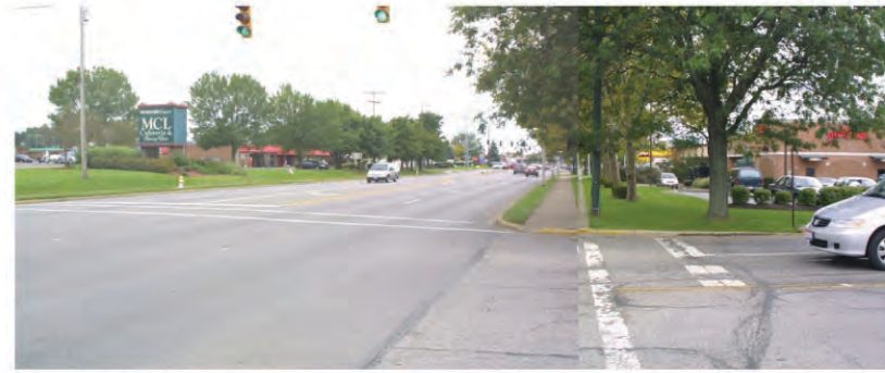
INTERSECTION OF WESTERVILLE SQUARE & S. STATE STREET (SOUTH VIEW)
