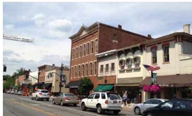
HEAVY TRAFFIC CAN CREATE UNPLEASANT, AND POTENTIALLY UNSAFE, CONDITIONS FOR PEDESTRIANS
