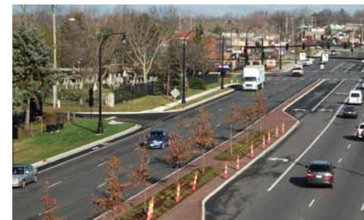
STATE ROUTE 3 IS A MAJOR NORTH-SOUTH CORRIDOR IN WESTERVILLE.
