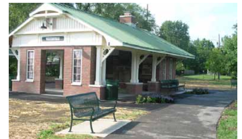
CREATING CONNECTIONS TO THE NEW BIKE DEPOT WILL HELP UPTOWN BECOME A REGIONAL BICYCLE HUB
