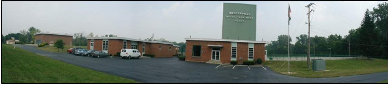
Figure 2. The City of Westerville’s Water Treatment Plant.
