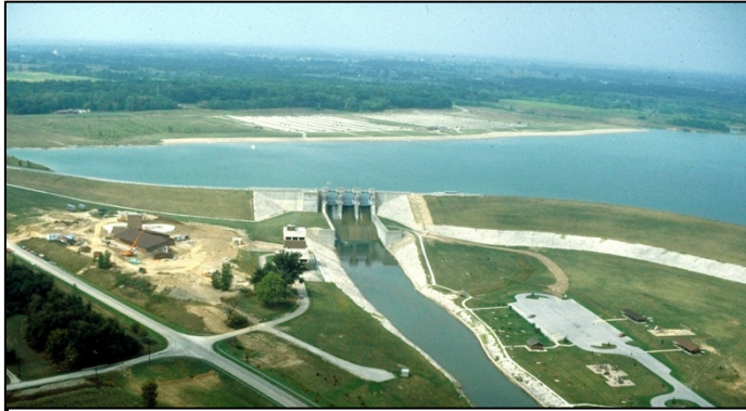
Figure 5. Alum Creek Reservoir and Dam, Looking Northwest.
