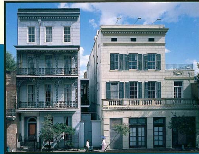
The same two buildings, 1993
