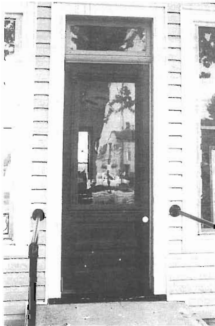
This Uptown Westerville door is a good example of late 19th and early 20th century practice. Note the paneling, ornamental treatment, and large glazed area.
