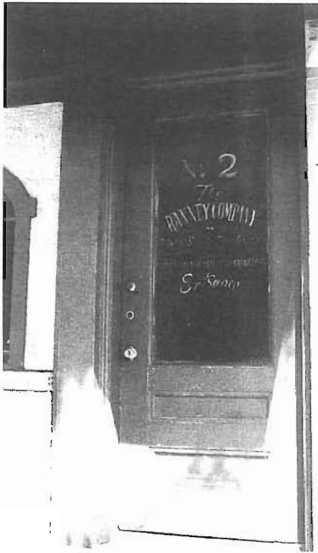
A typical late 19th century commercial building door, in this case serving as an entrance to an upper floor. Panels were common on such doors, but, unlike this example, they often had no glazing at all.
