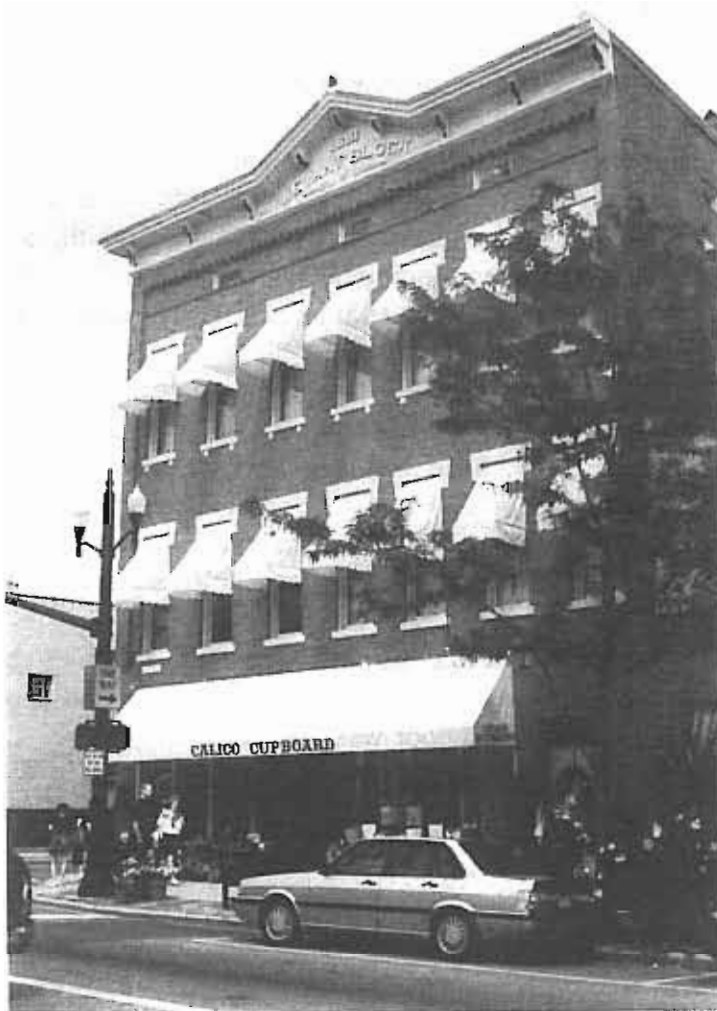
The Weyant Block, an Uptown landmark, illustrates the traditional use of both storefront and upper-floor awnings.
