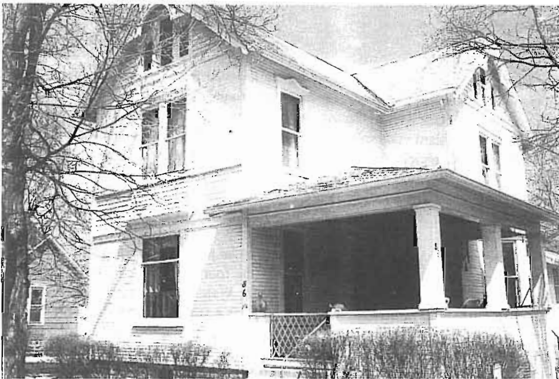
This Uptown Westerville home, which is of frame construction, retains its original wood siding and decorative features, including shaped rafter ends, cornerboards, window and door trim, and a simple but roomy porch.
