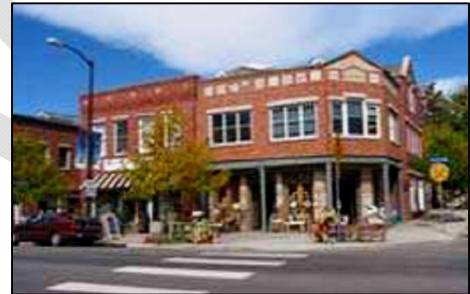
Example of appropriate massing and building materials
