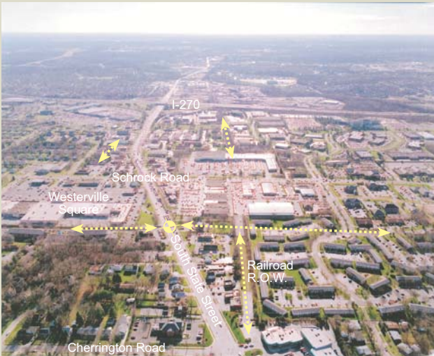
View south along S. State Street from Cherrington Rd.
