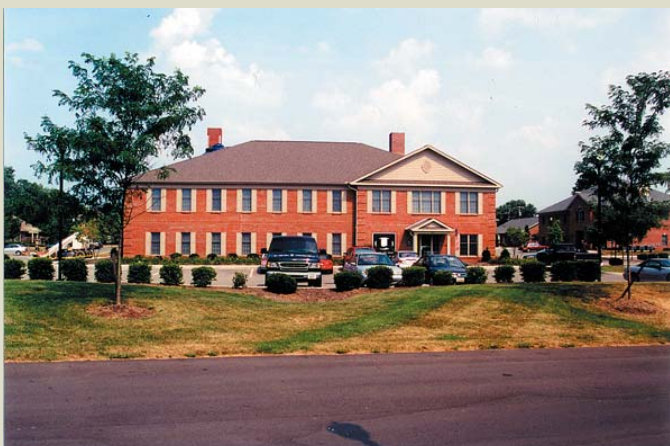
Two story structure
