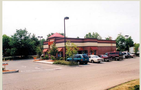
Primary and secondary exterior materials
