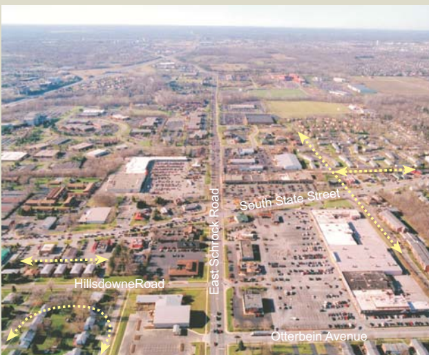
View west along Schrock Road from Otterbein Ave.
