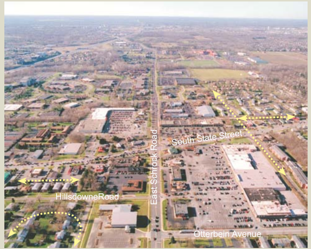
View west along Schrock Road from Otterbein Avenue
