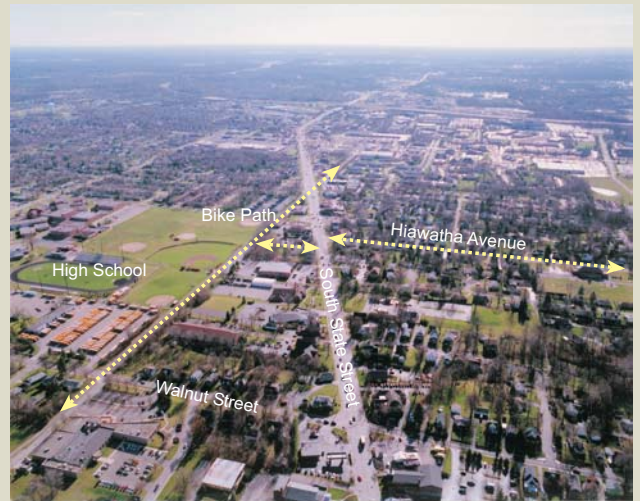
View south from Walnut St.
